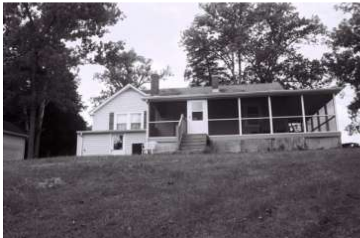
Photo 3: River Cottage, Rear (North) Elevation
