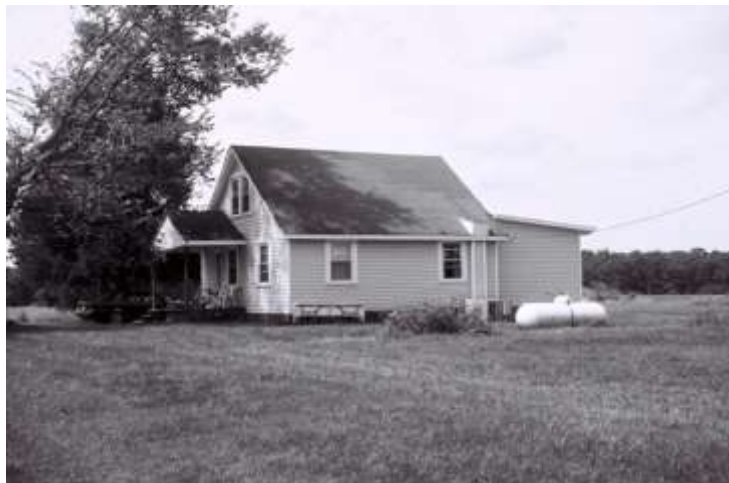
Photo 33: Hite House, Northeast Oblique View, and Propane Tank
