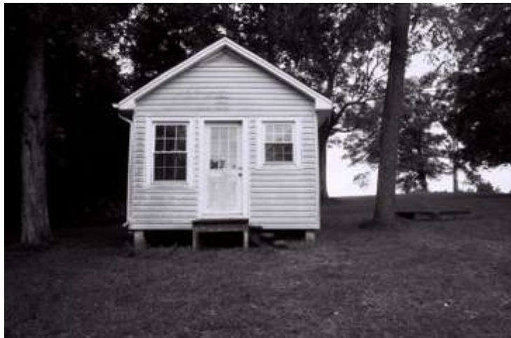
Photo 6: Servant's Quarter's, Front (North) Elevation
